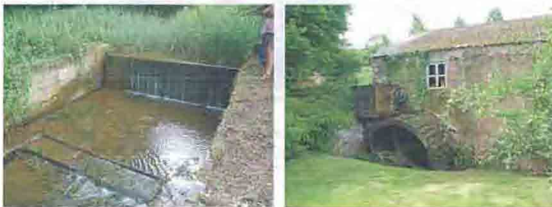
Figures 4.19 and 4.20. Gatcombe Mill pond dam and waterwheel, July 24 2008.
