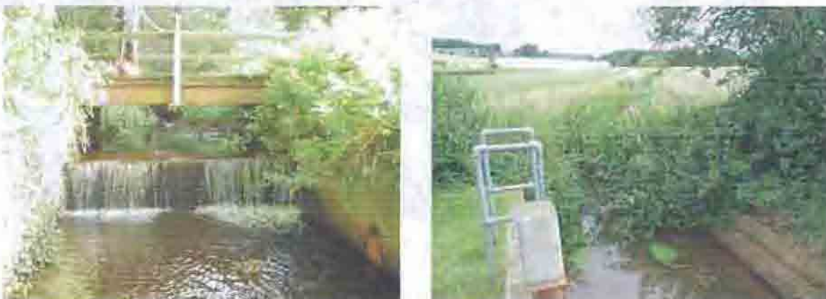
Figures 4.21 and 4.22. Left; structure 18. Right: structure 20, looking upstream.
