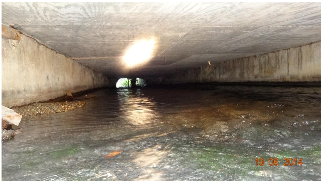
Figure 4: Cedar Hill Culvert
